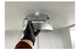
Slide the canopy up to meet the ceiling plate.
