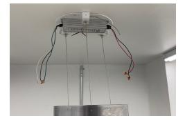
Pass suspension cables through grommets in canopy and lock into cable grippers in ceiling plates.
