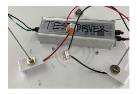
Ensure powered suspension cables are fully insulated inside the canopy.
