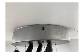
Fasten the Canopy in place with provided button head screws.
